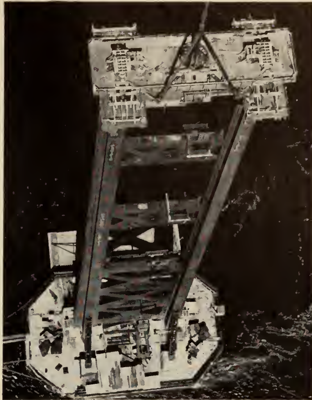
Aerial view of one of the 500 foot towers of the Tacoma Narrows Bridge at Tacoma, Wash.
